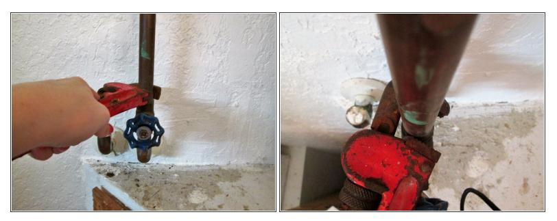
• Using a pipe wrench, detach all remaining pipes from the tank.
