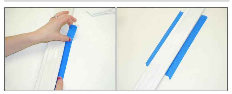
Tape the edges around the damaged area of the trim with masking tape.
