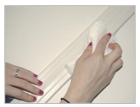
Wipe off the excess dust from sanding with a wash cloth.
