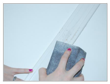
Sand down the damaged area of the trim using the block sanding sponge to make a smooth surface.
