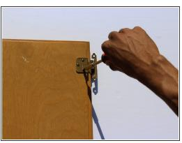
Place the new cabinet on a flat surface. Then line up the old (or new) hinge's to holes on the door.
