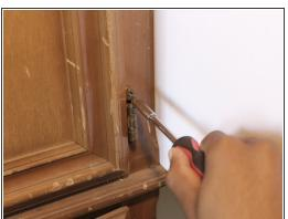
Finally, line up the hinge's holes with the holes from the previous cabinet door. Then screw the new door on.
