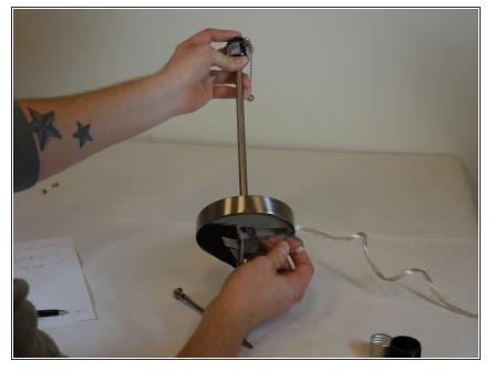
Position the socket/switch assembly on the base and pull the power cord from the bottom to set the socket in place. Reattach the felt or cork on the bottom of the lamp.
