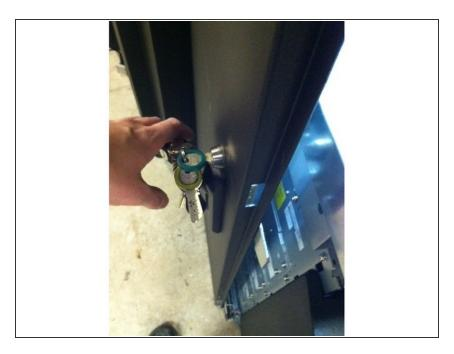
Make sure the door lock and handle are in good working order and not bent or loose
