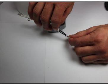
For each broken lightbulb, expose the wire leading to the bulb by pulling back the plastic coating on the wire while gently holding onto the bulb.
