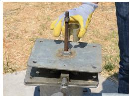
Remove the chain support from around the pump rod.
