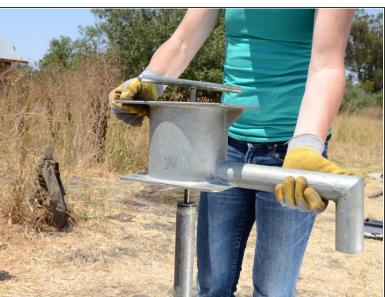
Lift the tank up a few inches above the top of the riser main.
