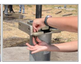
Secure the pipe vise to the top flange with two bolts and nuts to hold the pipe vise in place.
