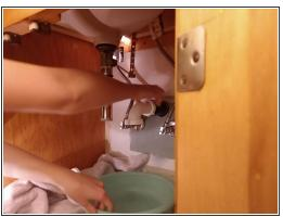
Insert the horizontal pipe back into the water output in the wall. Begin to tighten the nut closest to the wall.
