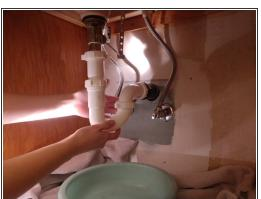
Loosen the coupling nuts from the pipe above and below the drain using a wrench.
