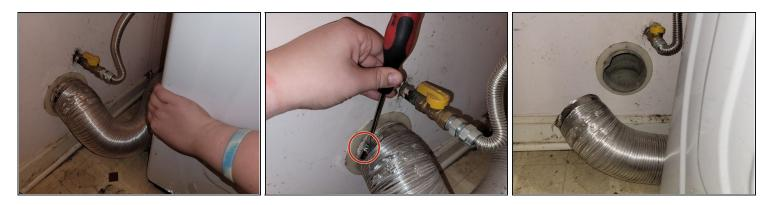
• Pull your dryer away from the wall and disconnect the dryer vent from the wall.
