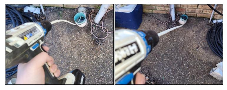
• Pull the cleaning extensions back out by continuing to run your drill in the same direction and pulling backwards.
