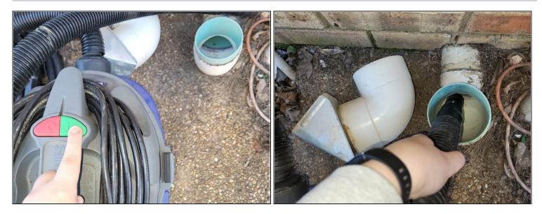
• Use a shop vac from the outside vent to remove any loose lint left behind in the vent.
