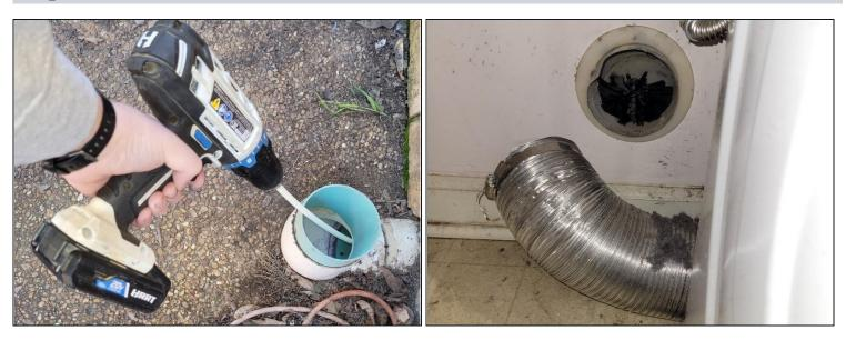
• Keep adding and running the extensions down the vent with the drill.
