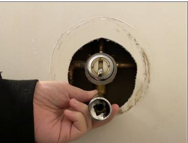
Insert the new diverter in place of the old one. Tighten with the deep socket or wrench.
