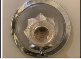
Reassemble the faceplate and knob. Remember to place the screws back in the places they were originally.
