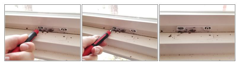
• Remove the left 12.7 mm screw on the lock keeper with a Phillips #2 screwdriver.
