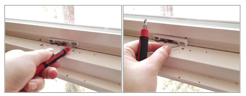
• Remove the right 12.7 mm Phillips #2 screw on the lock keeper.
