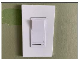
Attach the outer layer of the faceplate by putting it on top of the inner layer and slightly pushing it until you hear a click sound.
