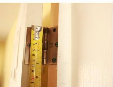
Take measurements of the door hinge using a tape measure and use the measurements to find a replacement door hinge.
