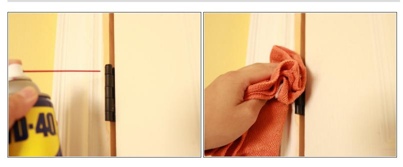
Spray a small amount of WD-40 at the back top and bottom hinge and wipe it down with an old rag.
