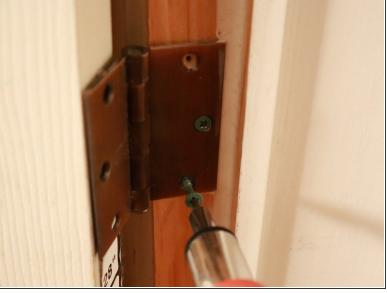
Repeat Step 3 with the bottom hinge on the door.
