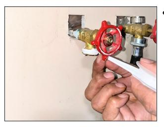
Wrap the new piece of Teflon tape around the shut-off valve connection.
