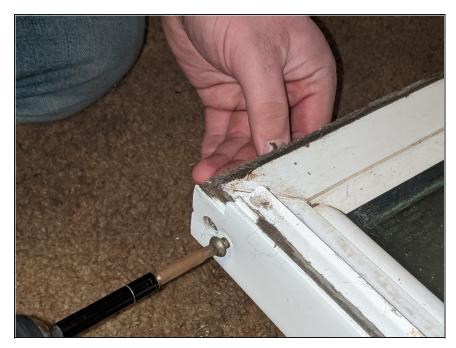
Using the Phillips #3, adjust the new rollers so they are at their highest point inside the door frame to easily put door back on tracks.
