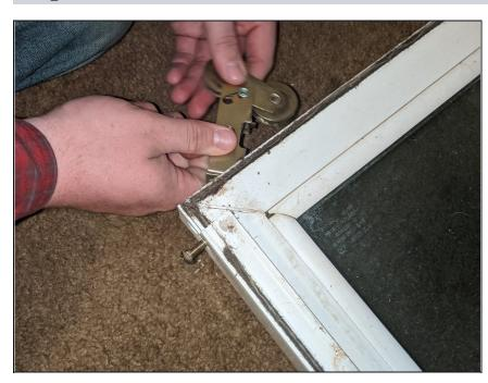
• Install the new door rollers by sliding them into place where the old ones were removed.
