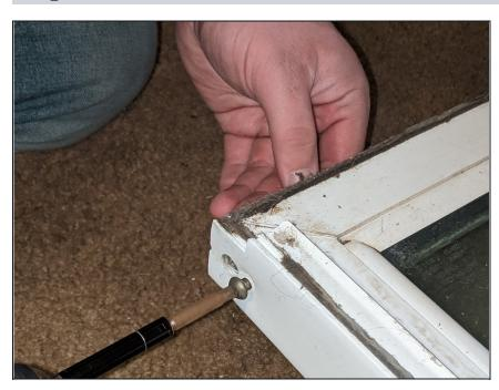
Place the doors on a steady table or surface. On the bottom of the doors near where the rollers are, there are two screws. Remove the top one with the Phillips #3 screwdriver to release the rollers.
