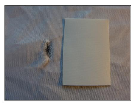
Trim the tape down until there is 1/2-3/4 of an inch excess on all sides of the tear.
