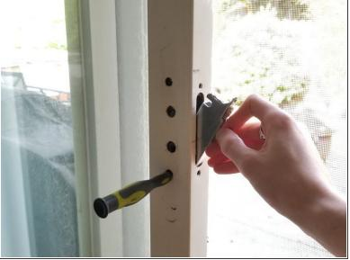
While holding the latch, move the mechanism downwards and remove it from the door.
