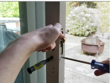
Using a Phillips #3 screwdriver, remove the two 13mm screws from the door while holding the latch.
