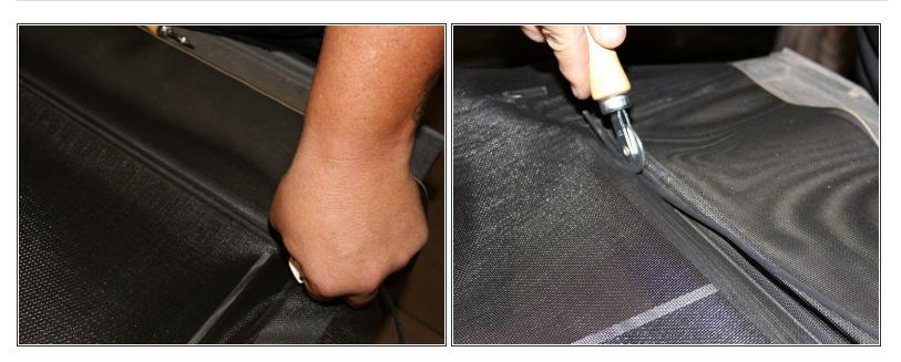
Begin at a top corner and press the spline down over the screen fabric and into the groove on the frame using the convex roller.
