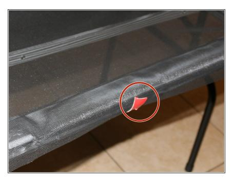
Tape or secure screen to prevent movement during spline installation.
