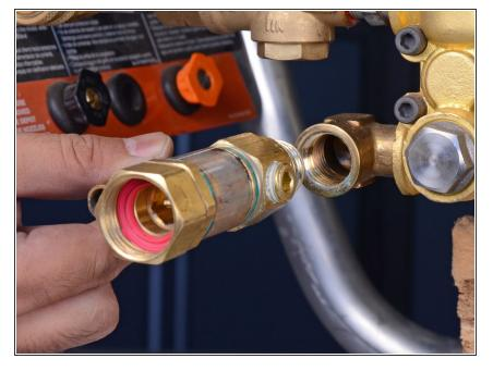
Remove the filter with the return elbow attached.
