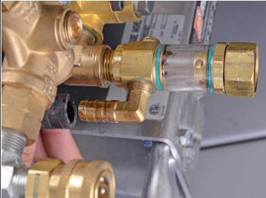
Wiggle the hose and pull it off of the brass nipple.
