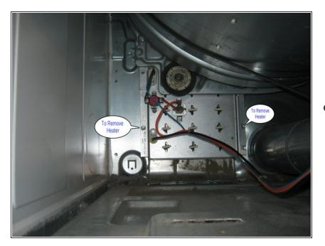
3) At this point you can see the heating element in the back lower left corner. Make careful note of
