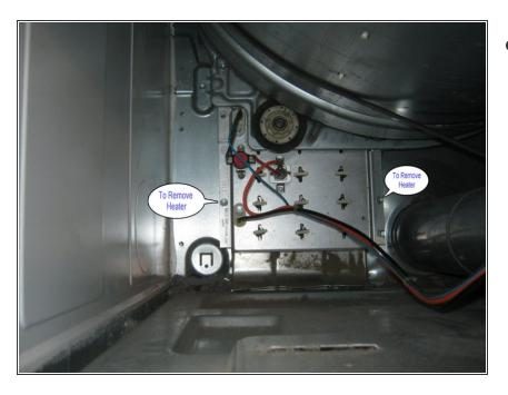
4) Remove the 3 wires (one 12ga black, one 12ga orange, one 14ga bl/bk). Check the resistance across the heater terminals - it should be around 10 ohms. Also Check for burned connectors.
