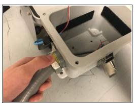
(i) Pull the wires through the connector piece and then screw the conduit onto the connector
