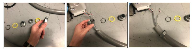
(i) Pull the cover over the conduit and the wires
