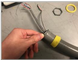
Pull this piece over the wires and then screw it into the conduit
