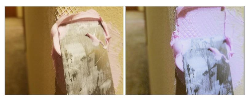
• Apply spackling paste over the mesh tape to fill the hole.
