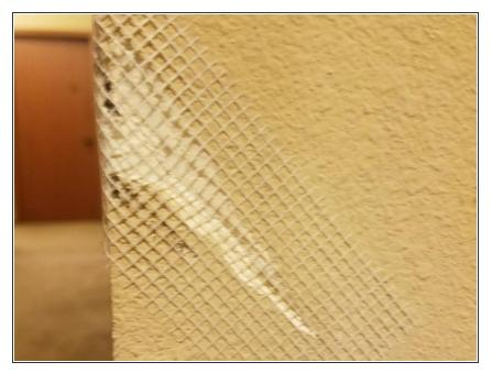
Apply a single sided mesh tape used for patch work to increase the strength of the material.
