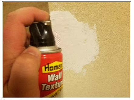
• Spray aerosol wall texture over the leveled patch in a quick fluid motion from one side to another.
