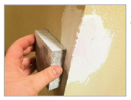
Sand the rough edges of the spackling paste to smooth the surfaces until it is flush with the wall.
