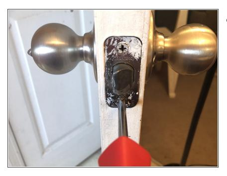
Use your screwdriver to tighten any loose screws found on the face plate.
