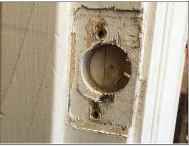
⚠ Use an electric power drill to remove the screws from your strike plate.
