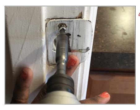
Using an electric drill, screw your strike plate into the wall.
