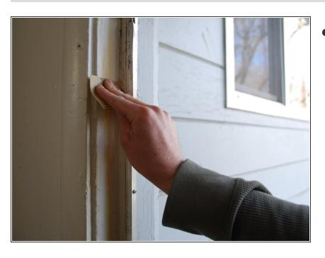
Sand the filled up cracks to get a smooth surface.
