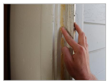
Apply wood filler into the cracks of the door frame.
